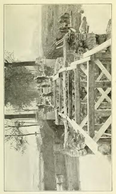
american engineers replacing a bridge at grand pré, three times destroute by shells
